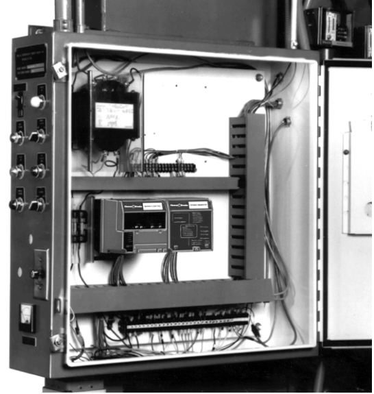
Fig. 5. Electrical panel installation.
