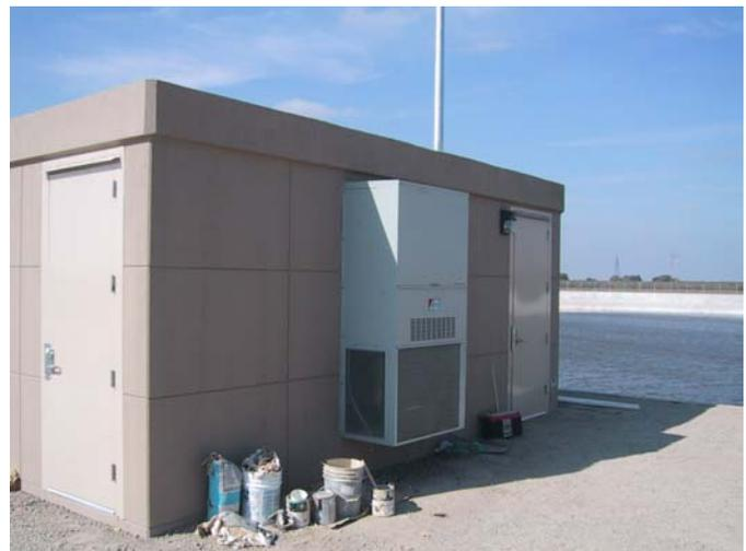
A new air conditioned enclosure for a VFD application at South San Joaquin ID.
